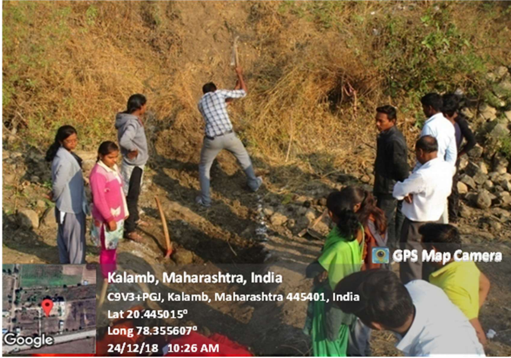
Snapshots During the Construction of Bund
